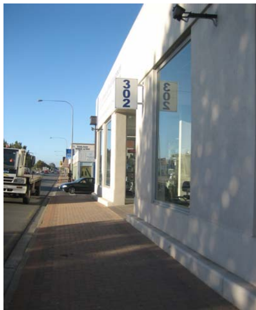
A view of our premises travelling south along South Road. Our premises are on the western side of South Road
